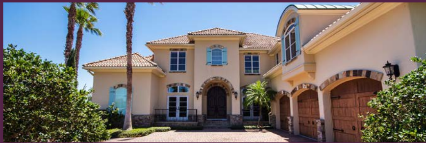
This private retreat in North Island at Marsh Landing has 3 acres of pristine land, 4 bedrooms and 4.5 baths. The unparalleled quality construction offers a gourmet kitchen, lanai and elevator. MLS# 881567 / $2,198,000
