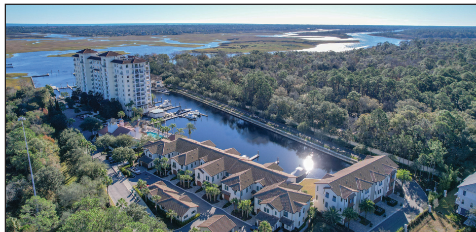
An aerial view of the condominium property.
