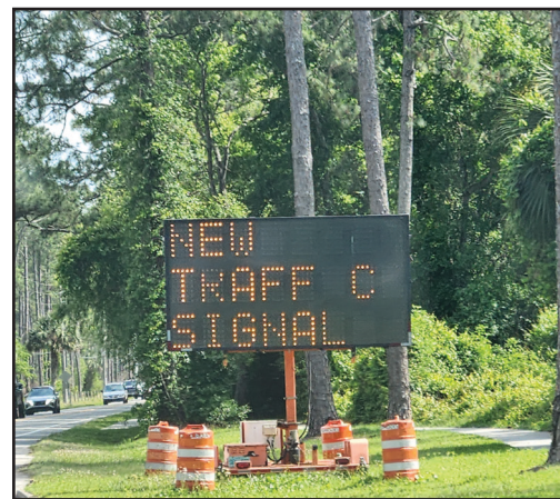
There are posted signs heading both directions along Palm Valley Road letting drivers know that the new traffic light is ahead.
