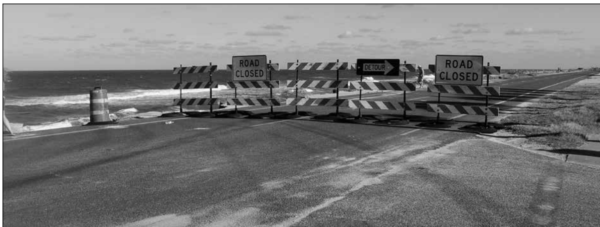
A1A was closed to traffic at the St. Johns County/Flagler County line, as Matthew washed away portions of the road.
