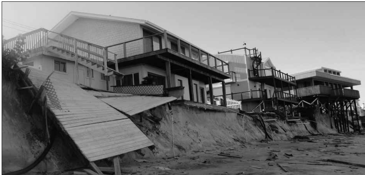
Extensive erosion have placed dozens of coastal homes in jeopardy.
