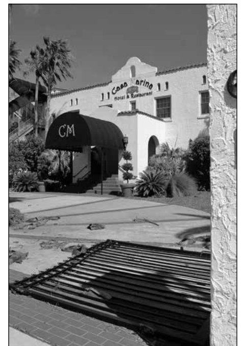
The historic Casa Marina Hotel sustained damage, including to its rooftop bar, but survived yet another storm.
