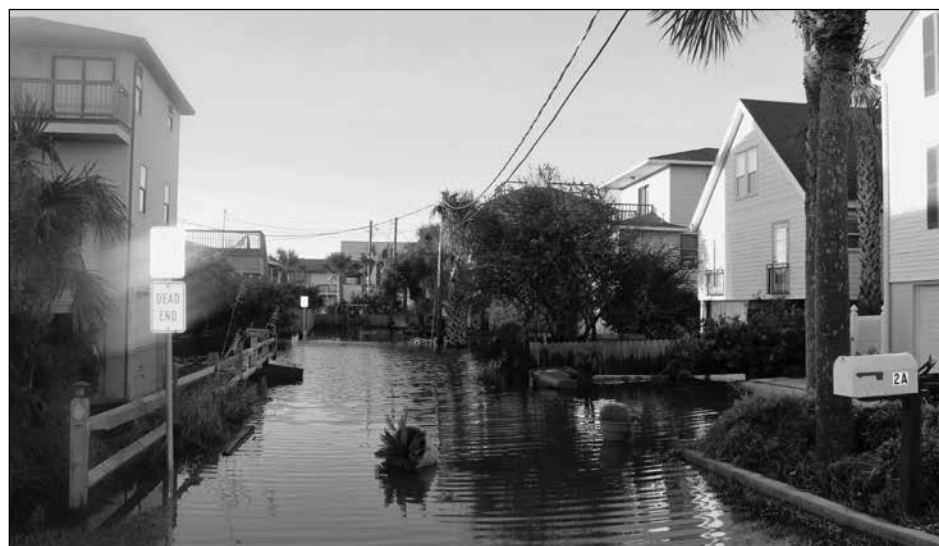
The Porpoise Point section of Vilano Beach suffered extensive flooding.
