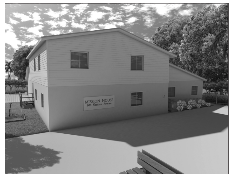
Photo provided by Mission House
