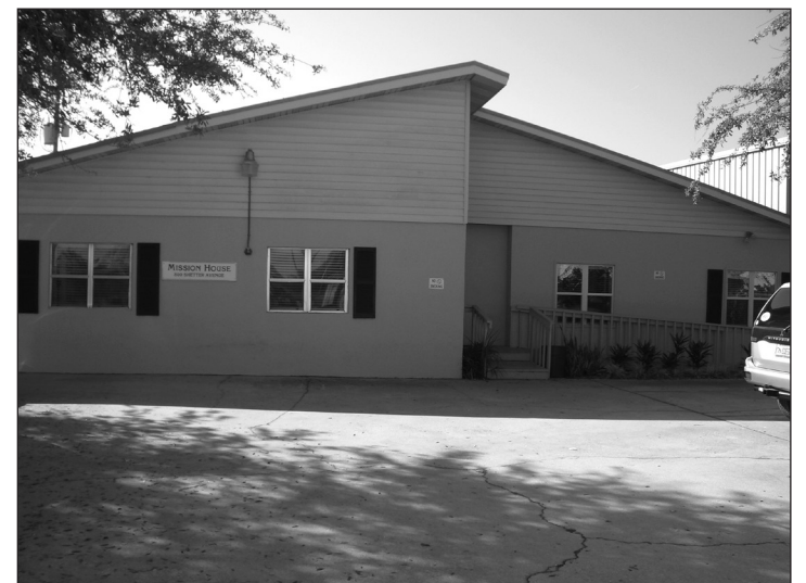
Photo provided by Mission House
