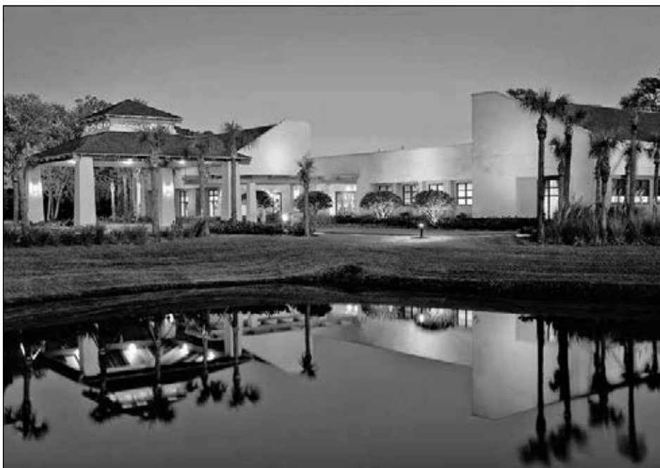
Sawgrass Spa Exterior
